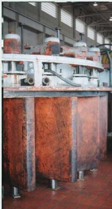
**Thordon SXL wicket gate and linkage bearings installed at Cameron Falls, Ontario**
