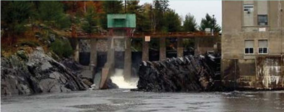
Frazzle ice is created when long periods of extremely cold weather, typically in the -35°C range, turn river water into a giant Slushie®. This isn't uncommon on The Spanish River in Northern Ontario, Canada, home of three Inco Hydropower Generating Stations. Frazzle ice is a regular occurrence almost every spring, pounding into the intakes and causing pumps that provide water to the turbines to ice up and shut down.
